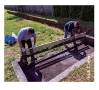
**Step 2:** Tap the screen against the inside of the sediment trap or use a broom/rake to remove material. Do this inside the sediment trap for easy cleanup.
