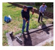
**Step 4:** Reinstall the trash screen. Dispose of material with regular trash.
