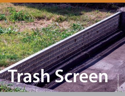
Make sure trash screens, also called debris barriers, are maintained annually so stormwater can flow through your facility properly.
